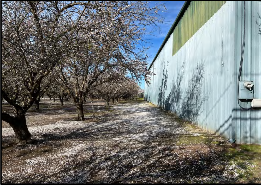
North edge of the site, looking west from the northeast corner of the site; 03/02/23.
