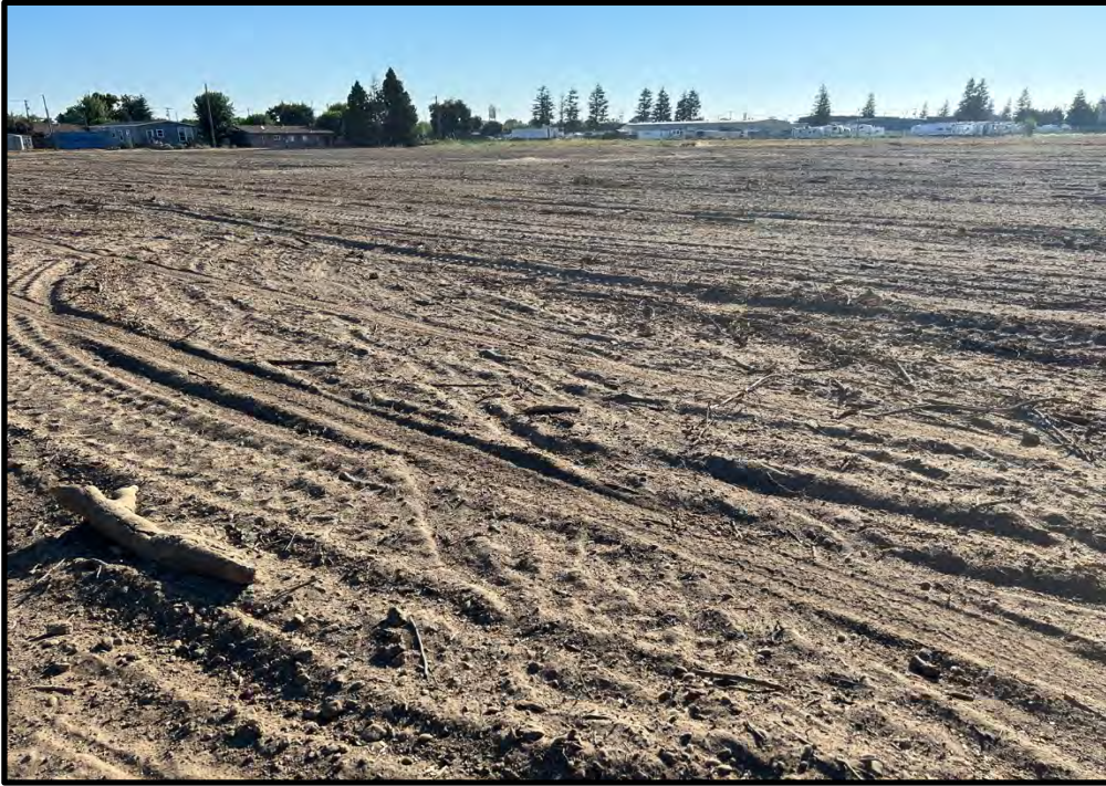
Body of the site, looking northeast from the southwest corner of the site; 07/07/23.
